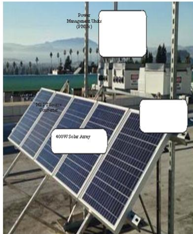
Fig A The scaled-down dc microgrid prototype used for ex-perimental validation.
